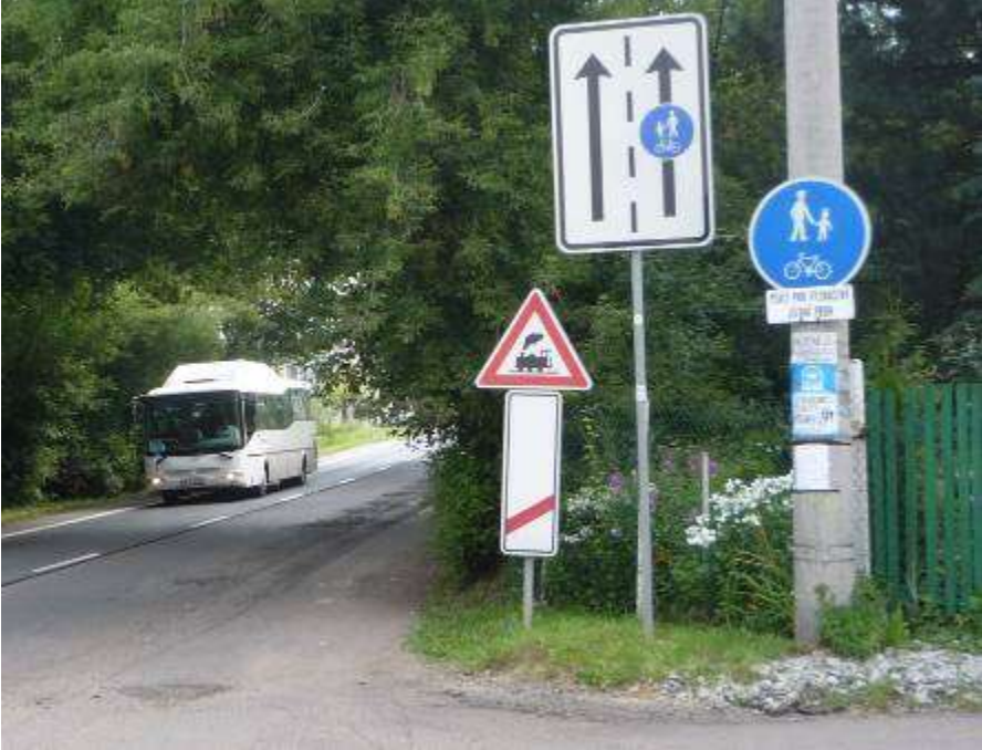
Figure 3.10 – Incorrect implementation of a pedestrian and cycle route
