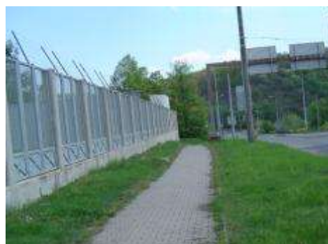
Pavement suitable for widening
