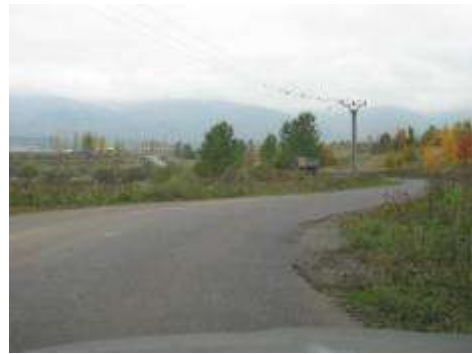
Road in the vicinity of the mining area
